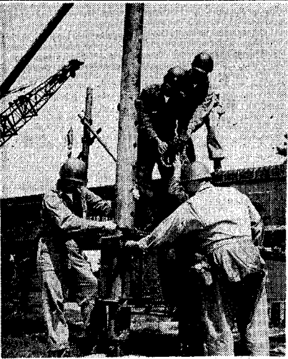
TIC ENGINEER TRAINING . . . U. S. Army Reservists of the Engineer School, Columbia, S. C., work on a road-way section of an engineer floating bridge during 15-days of active duty here. Lt. Col. William F. Stratton, left, and Lt. Col. H. C. Tysinger, right, both of Miami, Fla., tighten an upright section. Standing on the bridge-work are First Lt. F. N. Craver, left of Fayetteville, N. C., and Major Milton Klein of Mobile, Ala.
