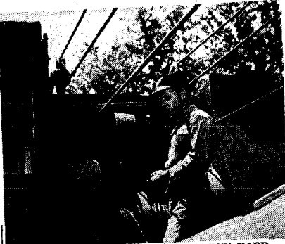
GIANT CRANE REPAIRED AT 'JUNK' YARD Sfc. W. D. Arnold Examining A Part
