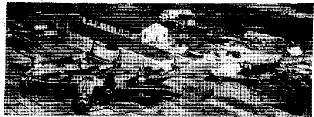
C-119s LIE CRIPPLED NEAR FLIGHT LINE AT LAWSON AFTER STORM'S FURY. Winds Tossed Flying Box-Car At Right Atop Several Gasoline Trucks
