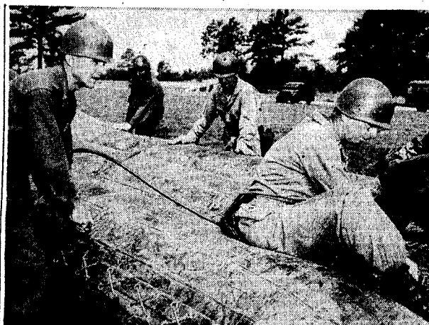
ENGINEER SCHOOL . . . U. S. Army Reservists inflate pontoons for a floating bridge erected during 15 days of active duty at Fort Benning. Left to right are Major Emyric Harris of Miami, Fla., Capt. H. A. Black of Charleston, S. C., Major Frank C. Houpt of Atlanta, Ga., and Capt. Everett L. Stewart of Tuscaloosa, Ala., all of the Engineer School, Columbia, S. C.
